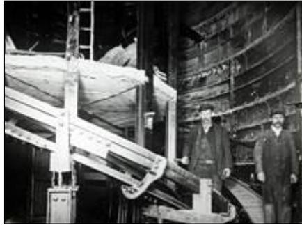
Lost spiral escalator at Holloway Road Underground station, 1906
